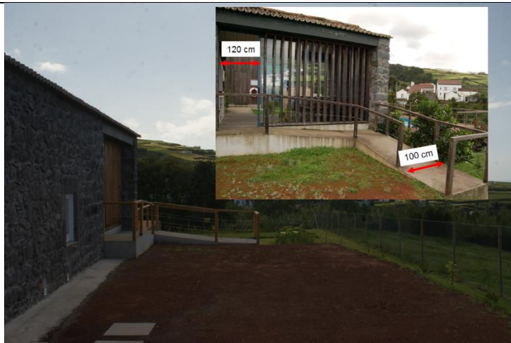
The private car parking with automatic car gate and the wheelchair ramp
